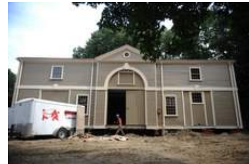
Workers with Geddes Building Movers on Tuesday prepare to move Gore Place's Carriage House to another location on the property. Wicked Local staff photo / Kate Flock
