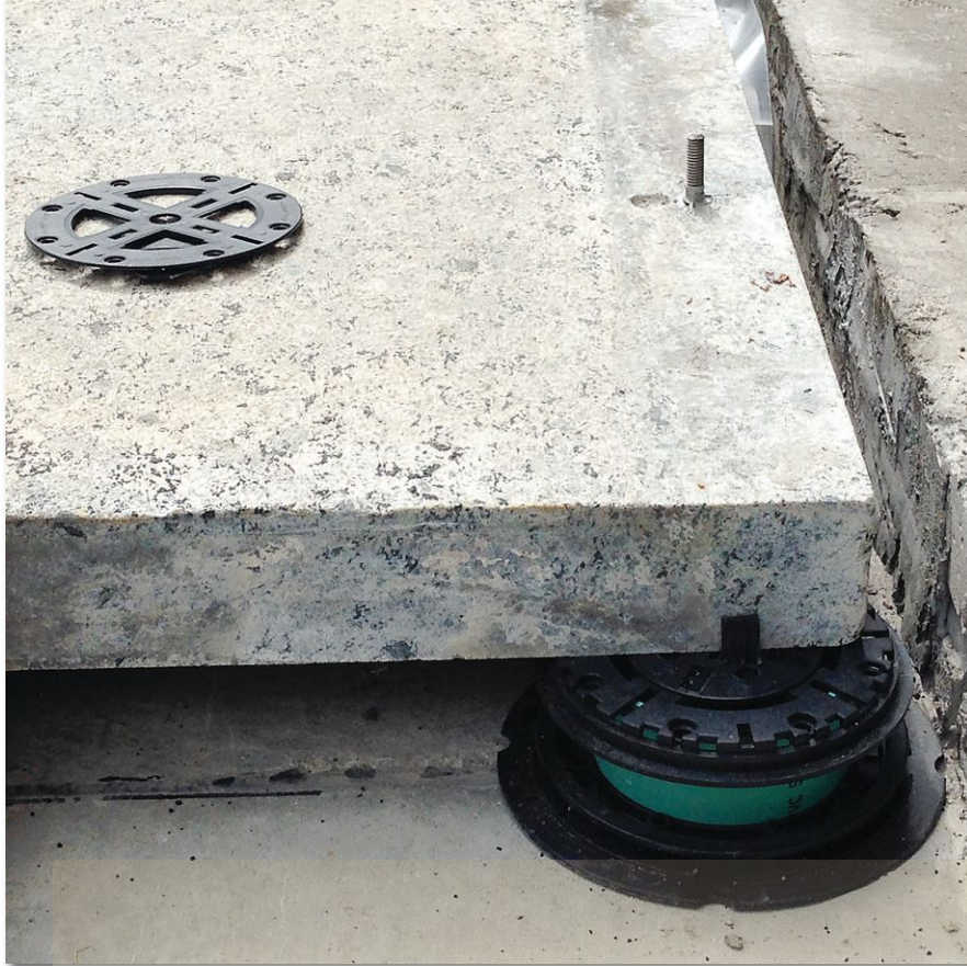
Existing stone was reset as a rainscreen using customized pedestals and hidden anchor components to improve drainage performance and reduce maintenance.
