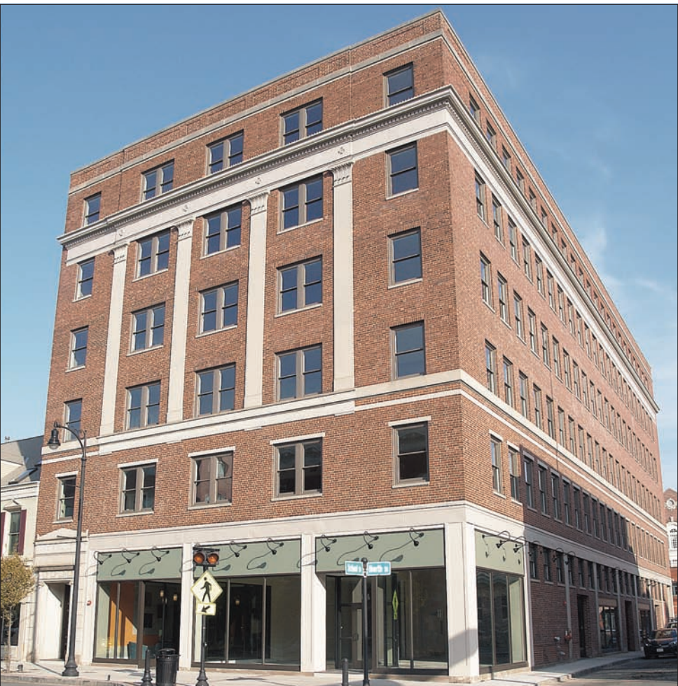
The upper five floors of the Onota Building have been converted into 25 upscale one- and two-bedroom apartments, known as Onota 74 Residences. The street-level space is being leased for commercial use.
