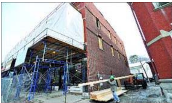
A worker for Allegrone Construction Co. brings lumber into the interior of the Baird & Benton block.
