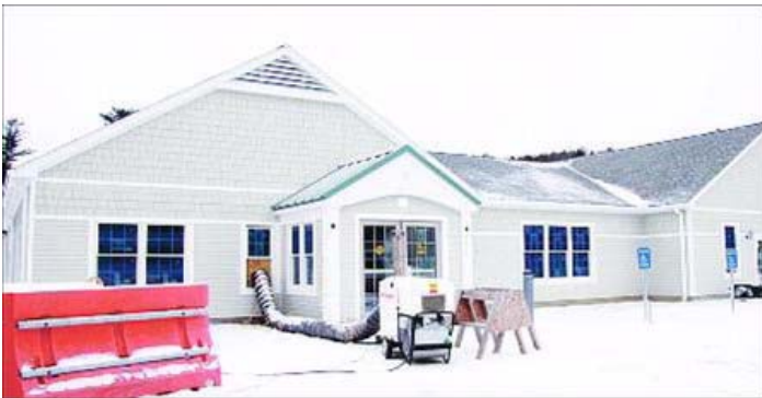
The new Dalton Senior Center is where the former Dalton High School used to exist. It should be ready for use not long after the start of the new year.
